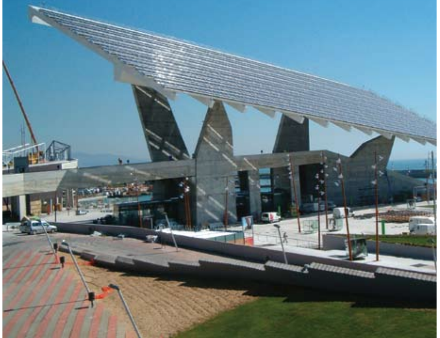
There are many applications which exist to integrate photovoltaic in buildings: here a semi-transparent module is integrated in a roof which also protects from direct sunlight (copyright: BEAR architects, M. van Kerckhoven)
